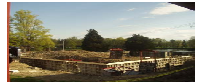
Construction on the New Provincial Offices
